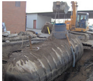
Underground Storage Tank Removal
