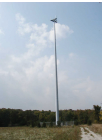
Cellular Tower Site Assessment
